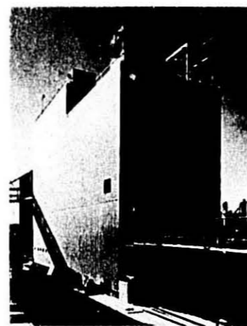
New Flour Mill—This free-standing windowless structure is International Multifoods' new milling facility at New Prague, Minnesota. Known as the New Prague "B" mill, the five-story 4,500 cwt. (hundred-weight) structure has an enclosed air system which filters air and provides a means of energy conservation through recycling. An insulated metal panel covers its slip-form concrete construction to meet energy conservation requirements.
